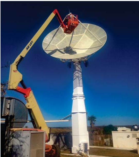
Radio telescope maintenance at the Learmonth Solar Observatory, Learmonth, Australia.
