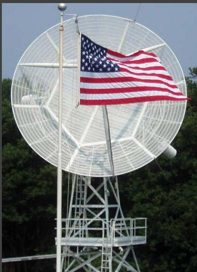
The U.S. Flag flies in front of an antenna located at the Sagamore Hill Solar Observatory. The Radio Interference Measurement Set antenna is 28 feet in diameter and a part of the Radio Solar Telescope Network, AN/FRR-95. Photo by Capt. Herbert Keyser.
